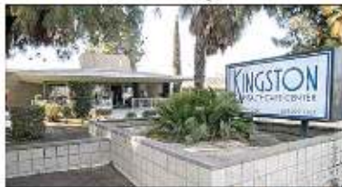
Real Road 4000 building facility Kingston HealthCare Center, shown in February.
