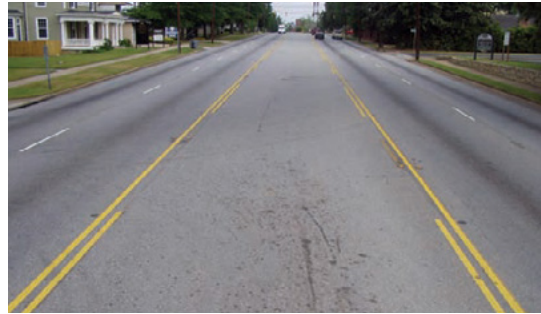
5 lane roadway with wide lanes, no bike lanes
