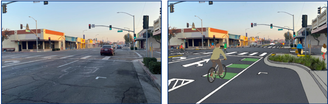
Figure 16: Bike Lanes at Yosemite Ave Between Lyons St & Mace St: Existing Design (left) vs. Proposed Design (right)
