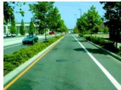
Reducing lane width can be both real (adding bike lanes and a median) and perceived (planting tall trees).
