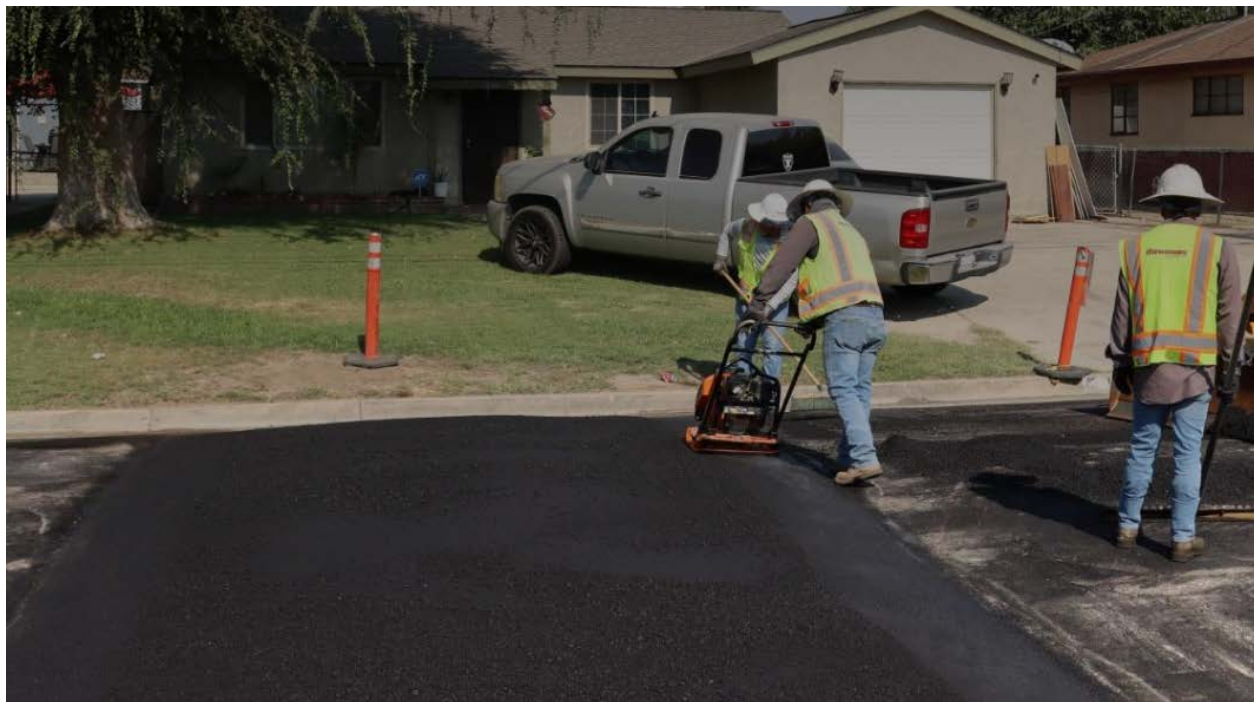
Photo of City of Bakersfield street crew installing a new traffic calming hump https://storymaps.arcgis.com/stories/23c4e43cdfdb424fb89be0d9c786ba9a
