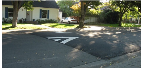
Picture of a speed hump located in a residential area. Photo from the Caltrans website
